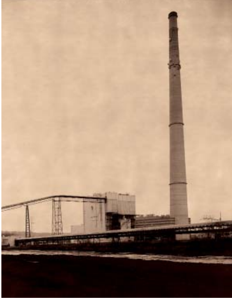
XCEL ENERGY'S ALLEN S. KING PLANT NEAR BAYPORT, MINN., IS ONE OF THE COMPANY'S MANY VALUABLE ASSETS.
